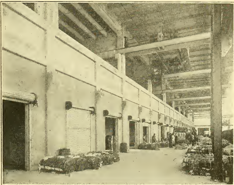
Interior View of Cotton Warehouse.
